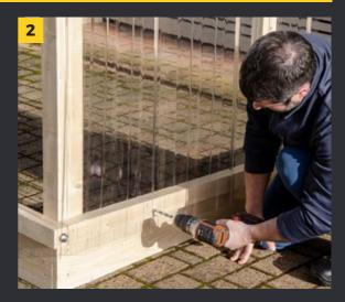
3 The holes (3 mm larger than the diameter of the screw) must be drilled with the sheets positioned correctly, especially at the overlapping points, where the holes must match perfectly. 4 In case of inverted installation, the length of the screws must be shorter than those applied on the roof; in fact, the corrugation of the sheet will be in direct contact with the structure of the wall.
