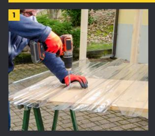
1 For the first row of sheets, holes can be drilled even before laying the sheets; this is quicker, but it is important to have taken the exact measurement from the free edge of the sheet to the first fastening batten, at the centre of which the screws must be inserted.
